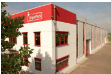
ErgoPack building in Lauingen: capacity created for further growth in 2010
