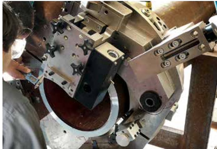
Nickel-plated High Speed Sever system, built to customer specifications, performs a critical role for rapid weld remediation on a pipelay vessel.
